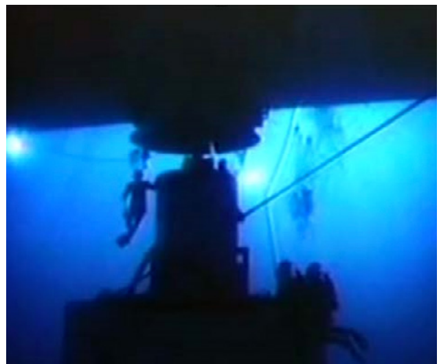
Figure 4.4 Vertical mating of the OTEC-1 cone CWP offshore Hawaii
