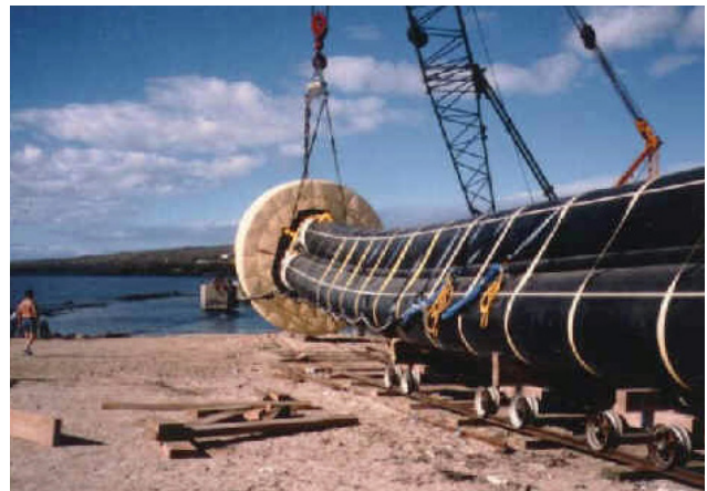
Figure 4.3 Horizontal launch of the OTEC-1 cold water three pipe bundle, Big Island of Hawaii
