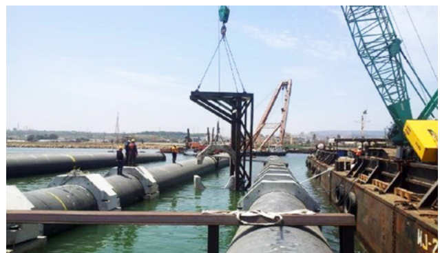
Figure 8.3 Concrete collars on a 2.5m water intake pipeline, Ras Djinet Gas Turbine Power Plant, Algeria
